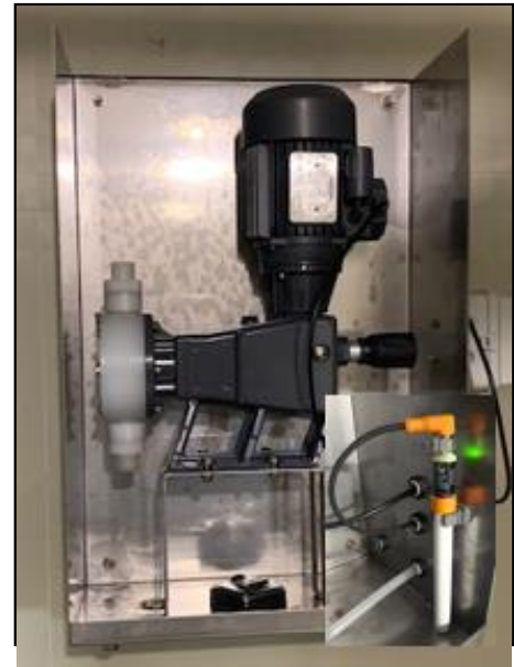
Figure 4: Sulphuric acid pump
